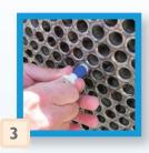
Insert tube plug all the way into tube until the collar comes to rest on the tube sheet.
