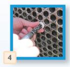
Holding the collar in place, use HEPCO pre-set torque wrench and torque down hex head nut.
